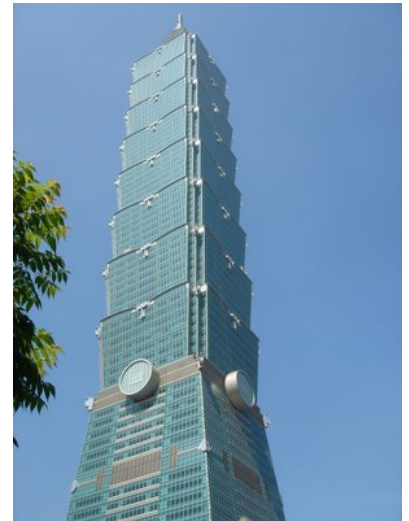
Taipei 101, Taiwan - The world's tallest building with 101 floors.
